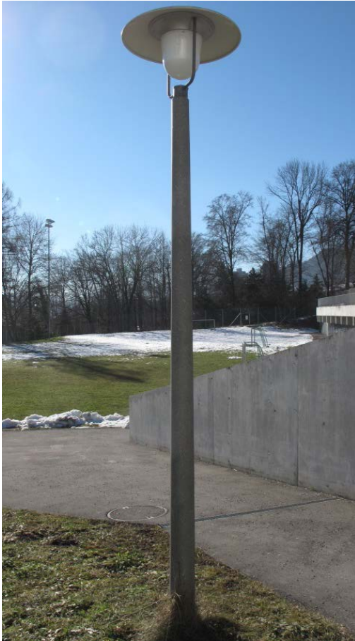
Figure 9: Centrifugally-cast, CFRP-prestressed HPC lamp pole; Location: Zurich, Switzerland.
