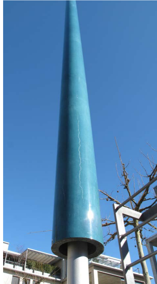
Figure 10: Slender, CFRP-prestressed HPC pole setup as a design element in a housing complex; Location: Uster, Switzerland.
