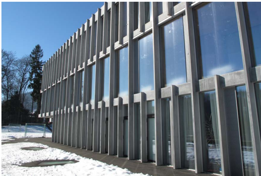
Figure 8: Building façade elements produced with CFRP prestressed HPC; Location: Zürich, Switzerland.
